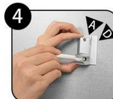
4. Align the first marked hole then mark the under hole
