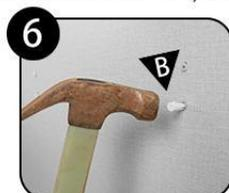
6. Use a hammer to drive "B" into the wall
