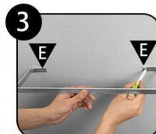
3. mark two top mounting holes(total four holes)
