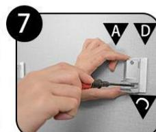
7. Use screw "C" to fasten the bracket to the wall from under hole
